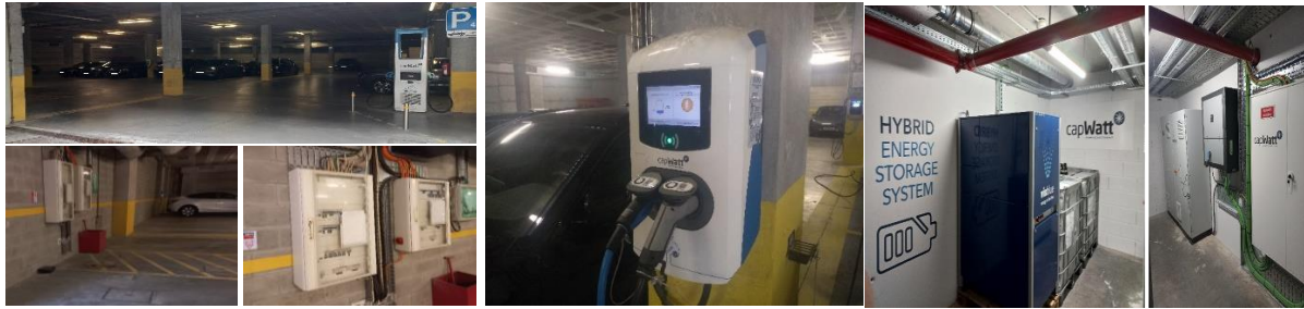
Figure 2 – EV charger detail and parking lot part of Use Case 6 (left and center), and Vanadium Battery from Visblue manufacturer and Lithium batteries, part of Use Case 5 (right)
