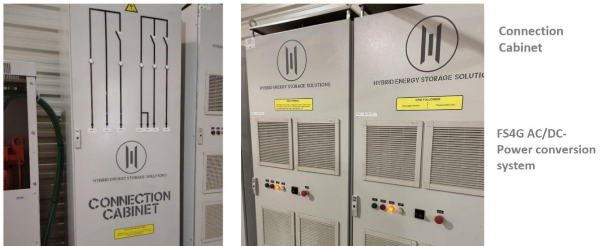
Figure 9 - Connection cabinets and power conversion system at HESS
