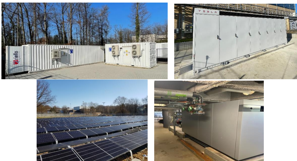
Figure 4 - Overview of assets integrated at Jülich Living Lab Energy Campus. From the top-left corner: Riello battery system, Tesla battery system, photovoltaic installation, heat-pump.
